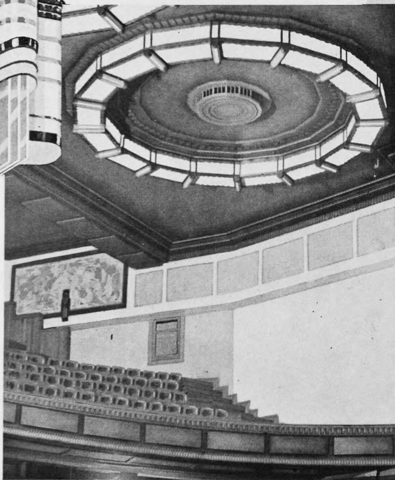
View showing ceiling fixtures.
